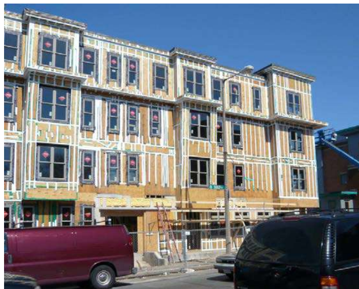
Figure 2.4. Dudley Village apartments under construction.
